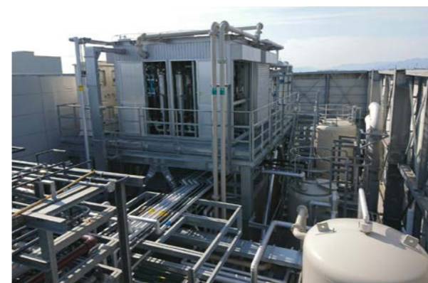
Kumamoto TEC's facility for recovery of water used for gas combustion treatment
