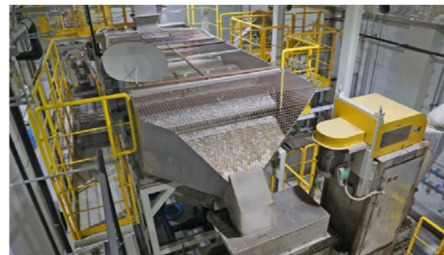
Equipment used for sink/float sorting, one part of the high purity sorting process at Green Cycle Corporation
