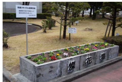
Flowerbed made from blocks of recycled sludge
