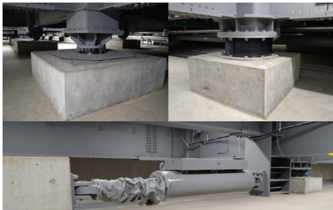
Hybrid seismic isolation structure
