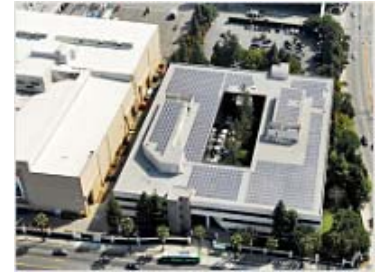
Solar power generation facility installed on the roof of SPE's headquarters
