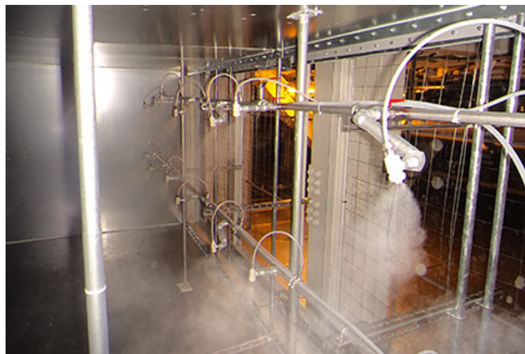
The two-fluid humidification system releases mist.
