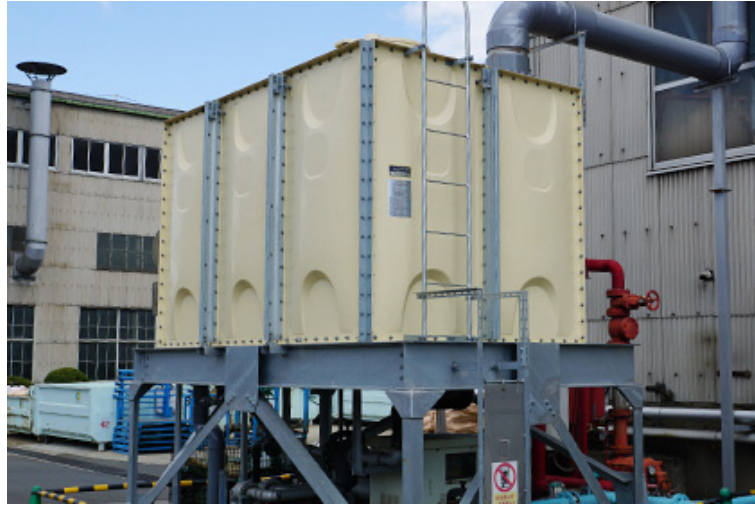
A rainwater storage tank next to the warehouse building
