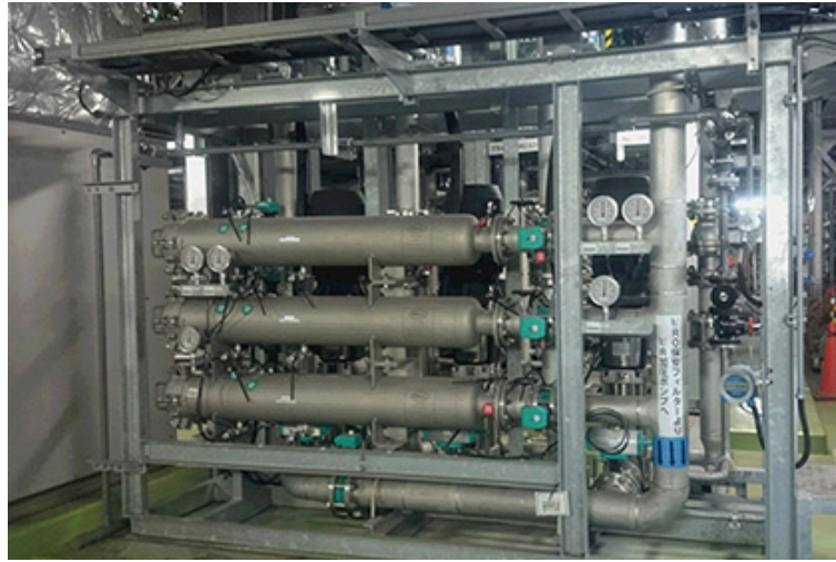
Blow water is reused for the reverse osmosis (RO) membrane filtration system.
