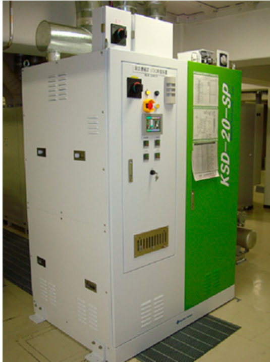
Small, fixed, condensing-type VOC treatment system developed by SCK in conjunction with an equipment manufacturer
