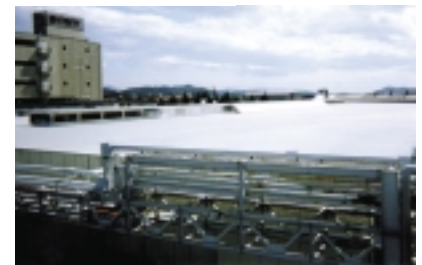
Reflective, insulative roof coating at Sony Motomiya
