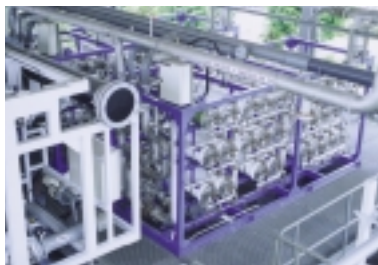
The water reprocessing system of Sony Display Device (Singapore)
